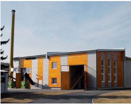
Heating plant Wieselburg
