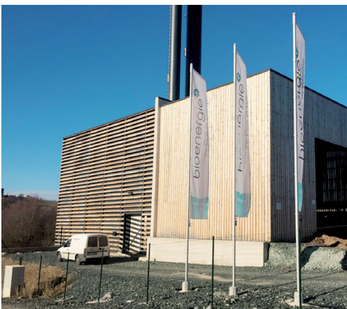
Biomass heating plant Stegersbach
