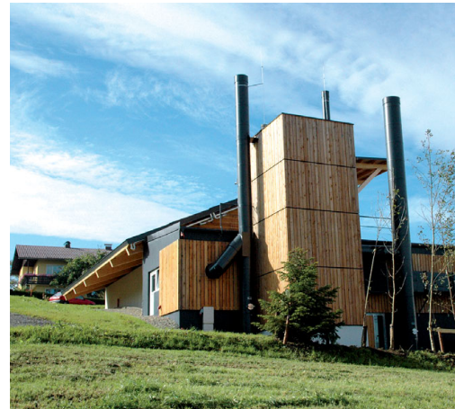
Heating plant Mattsee
