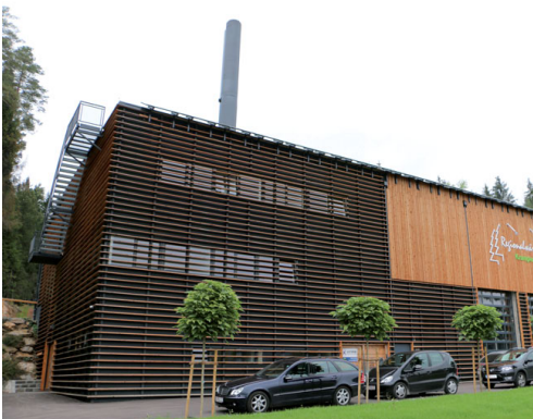
Heating plant Krumpendorf
