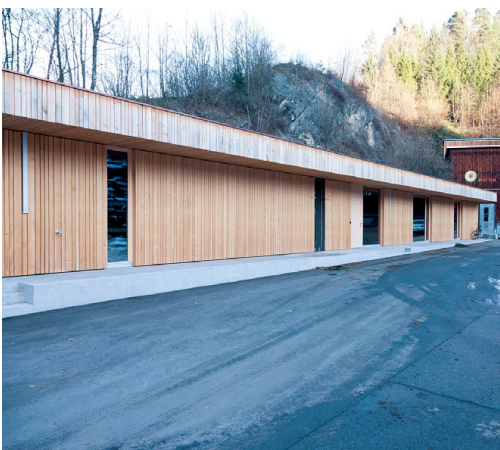
Heating plant Rankweil
