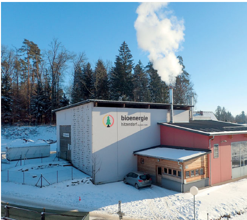
Heating plant Hitzendorf
