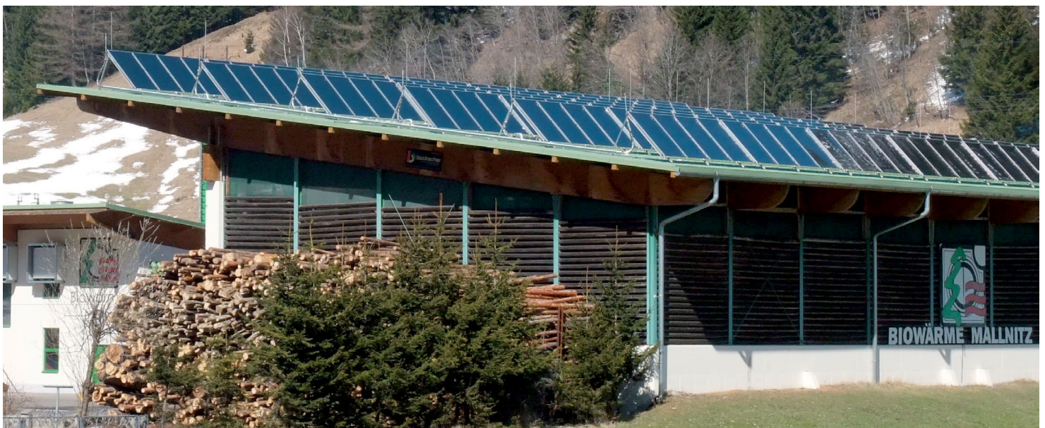
Heating plant Mallnitz
