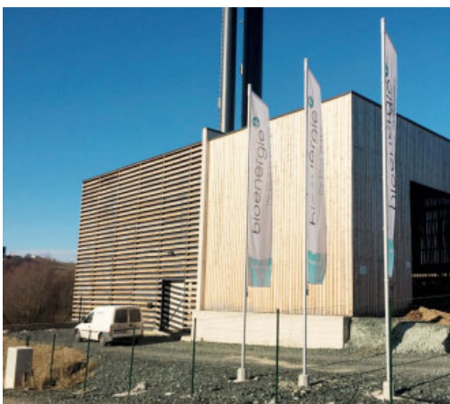
Biomass heating plant Stegersbach
