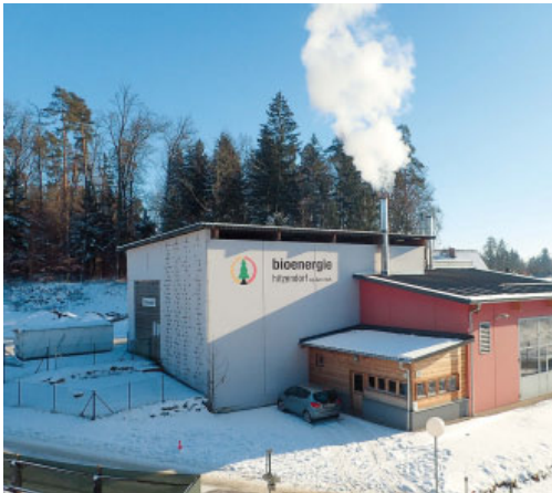
Heating plant Hitzendorf
