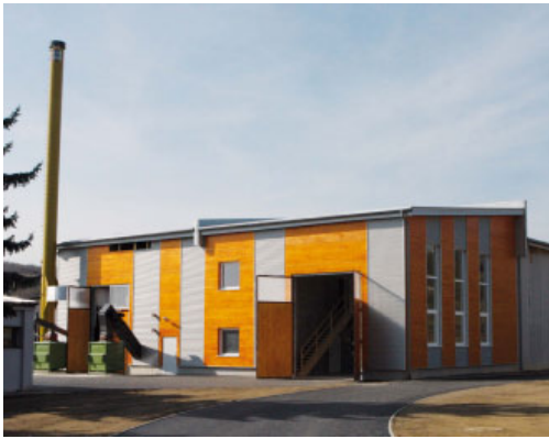
Heating plant Wieselburg
