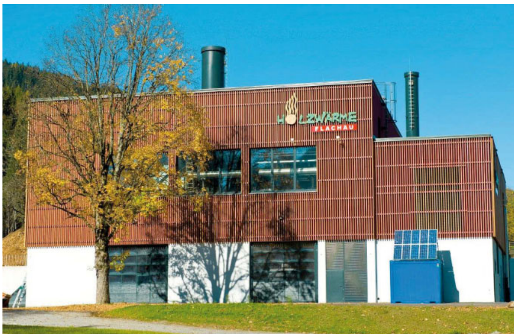
Heating plant Flachau
