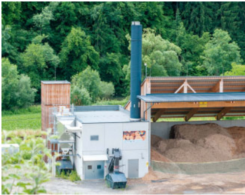
Heating plant Brückl
