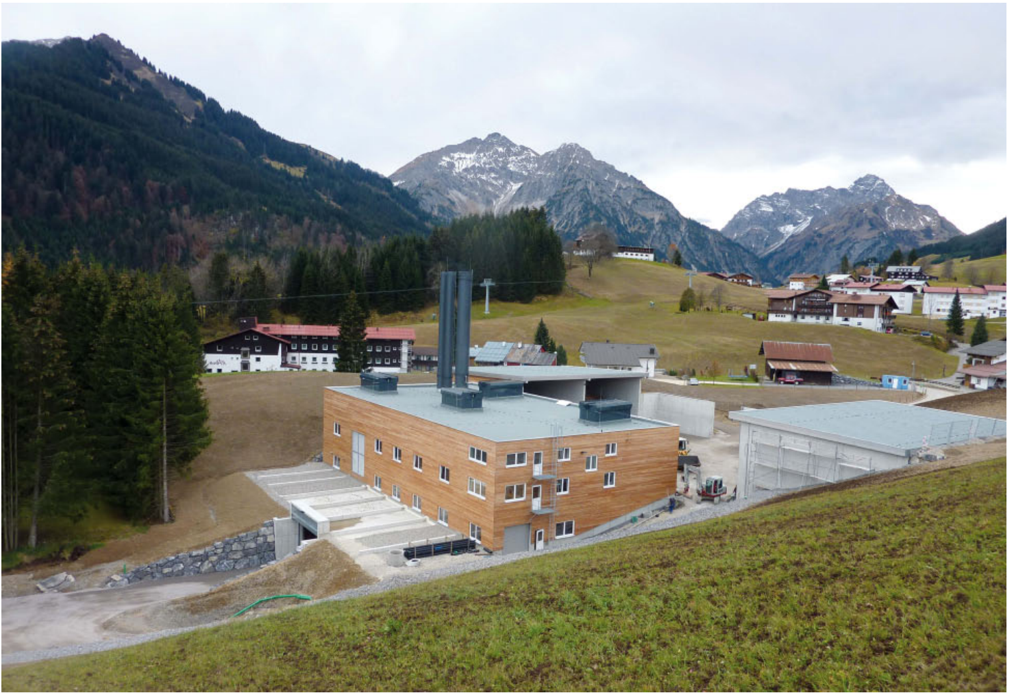
Biomass heating plant Kleinwalsertal
