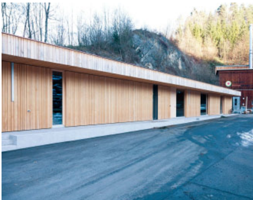
Heating plant Rankweil
