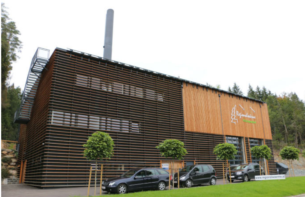
Heating plant Krumpendorf
