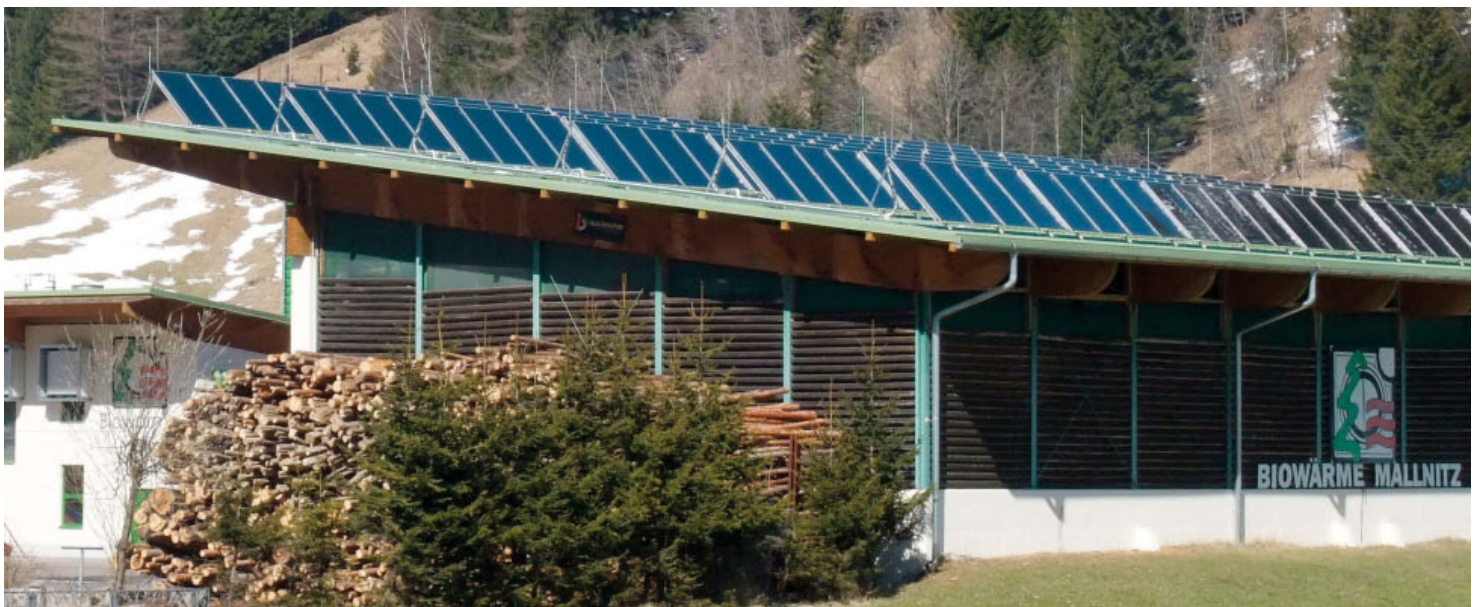
Heating plant Mallnitz
